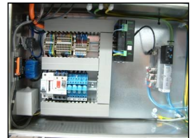
Switch cabinet detail
